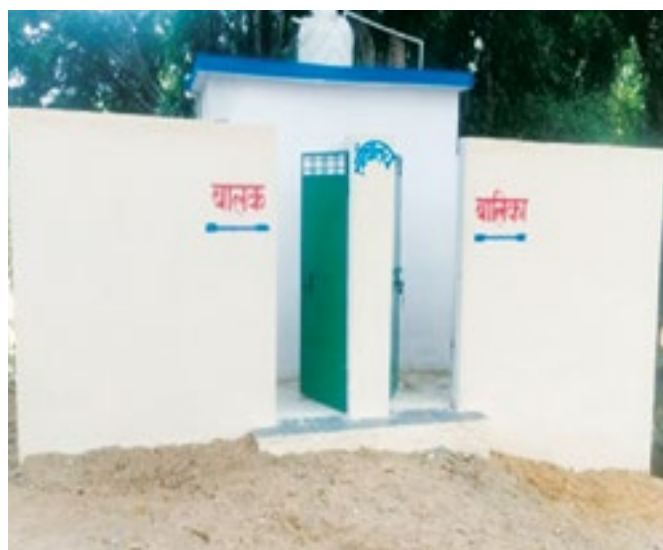
Toilet Block for School Children, Okhalgarah School, Dumri, Jharkhand
