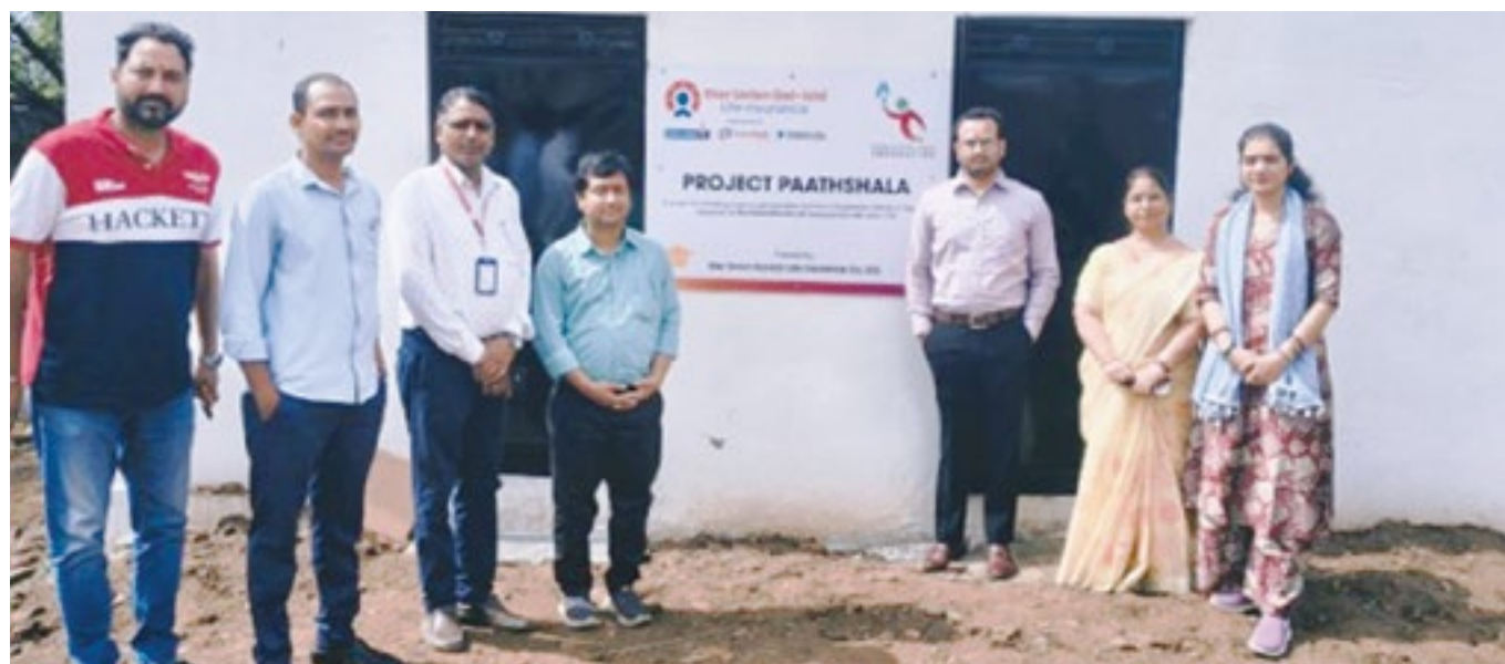
New Toilet Block at Jhor ZP School, Rajasthan
