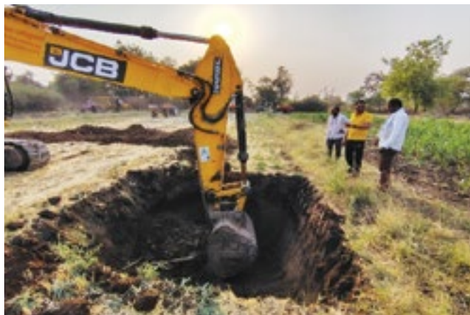
Water Recharge Pit (Jalkund)
